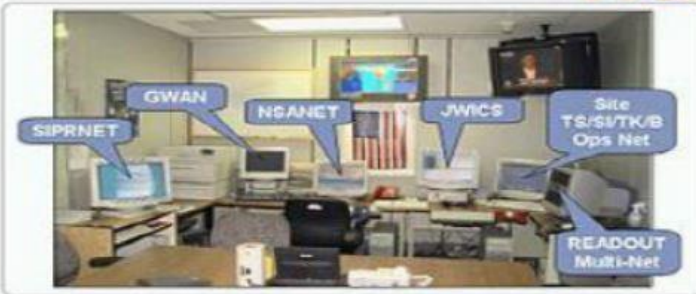
Behind the Green Door secure communications center with SIPRNET, GWAN, NSANET, and JWICS access
